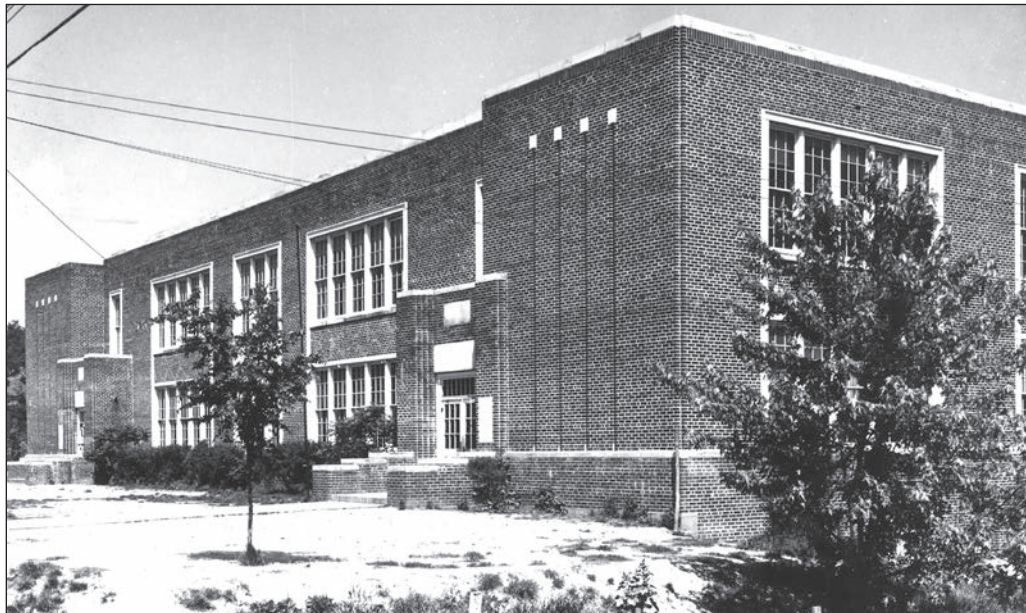
This is the Waynesville school building on North Street in 1950. It is the third school built on this site. The first was a frame building constructed in 1886. It was used until 1906 when a new concrete block building replaced it. It was razed in 1936, and this much larger WPA-assisted modern brick school was built. It even had indoor plumbing and a basement cafeteria, both absent in the old block schoolhouse. It served grades 6-12 until a new high school was built in West Waynesville. It then became a Junior High School (grades 6-9), and then a middle school (grades 6-8). It was razed and the Pulaski County Justice Center erected on the site in 2020.
